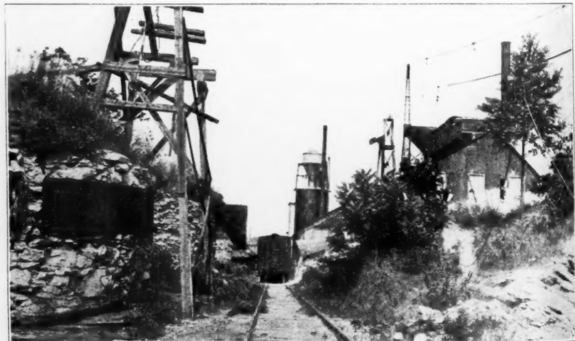
Railroad Spur Alongside the Plant
